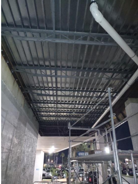
<-- EAST Canopy New Decking and Joists.
