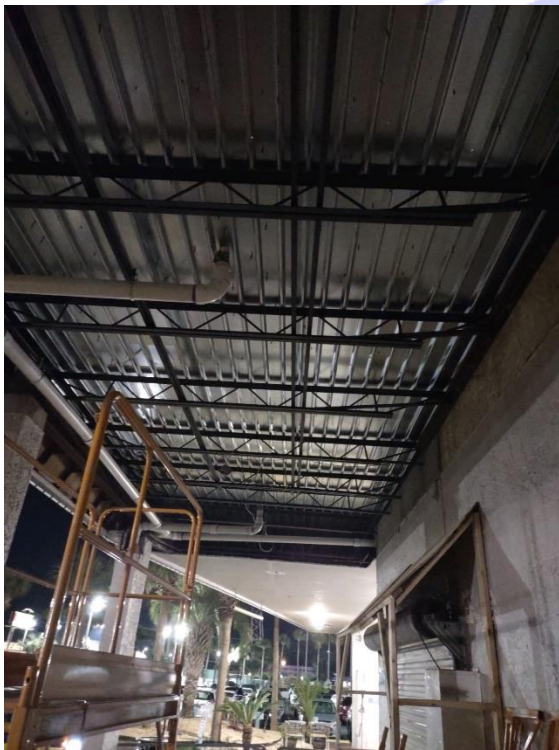
<-- West Canopy New Decking and Joists.
