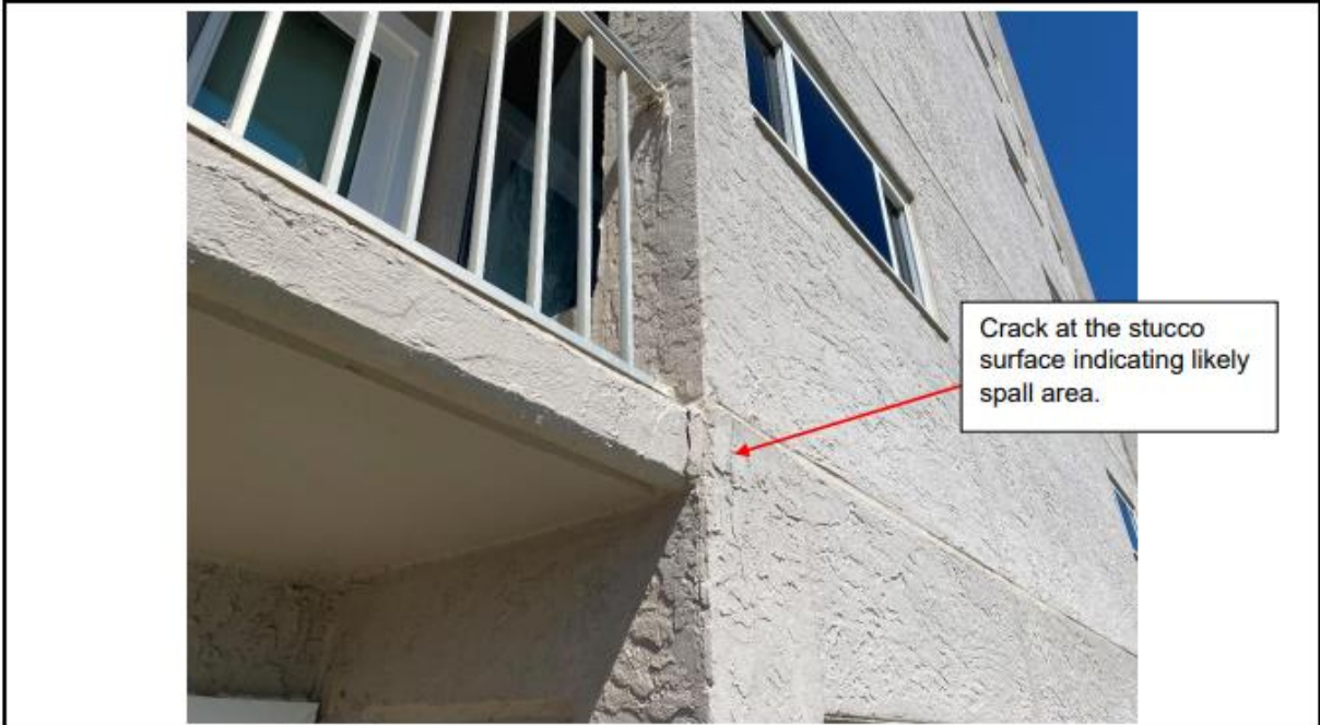
Photo 17 | Southeast Corner at 1 st Level
