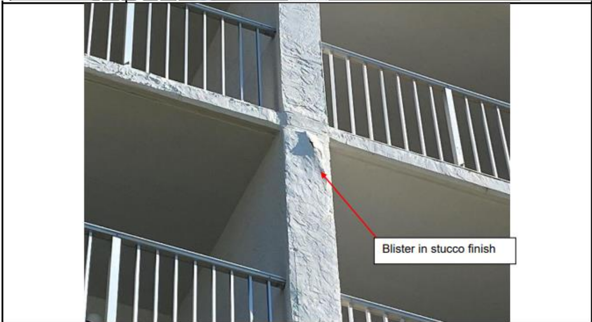
Photo 18 | Partition Wall Between Units 430 & 431
