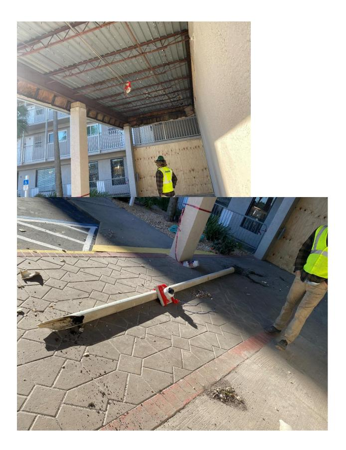
While the vendor was removing stucco, the drain pipe attached at the ceiling fell. The drain did have an excessive amount of debris inside. C Sharpe has contacted a plumber to schedule the repair. To be efficient and limit further issues, this will be repaired after C Sharpe completes the metal work in that area.
